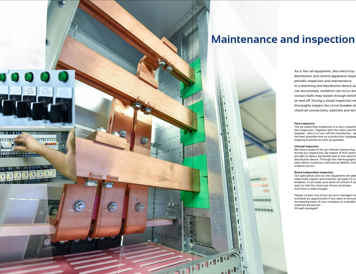
As in fact all equipment, also electricity distribution and control apparatus require periodic inspection and maintenance. In a switching and distribution device dust can accumulate, oxidation can occur and contact bolts may loosen through switching on and off. During a visual inspection we thoroughly inspect the circuit breaker and check all connections, switches and wiring.
